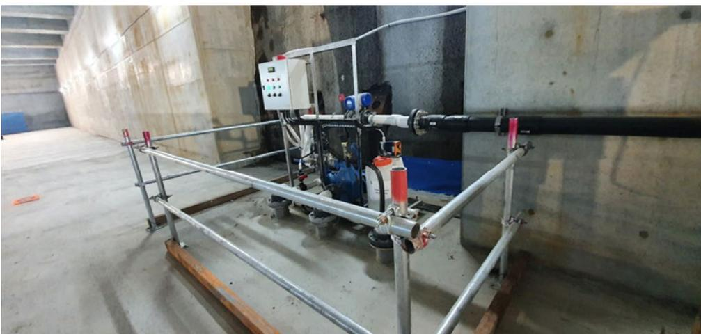
**Figure 4** B6 Sump at the base of the northern shaft (GW-2)
