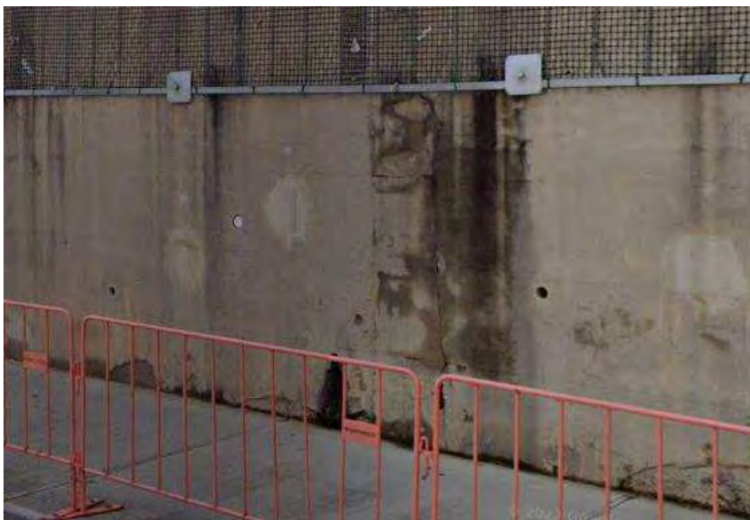
Figure 7: Cracking at the location of SBR 3.2.
