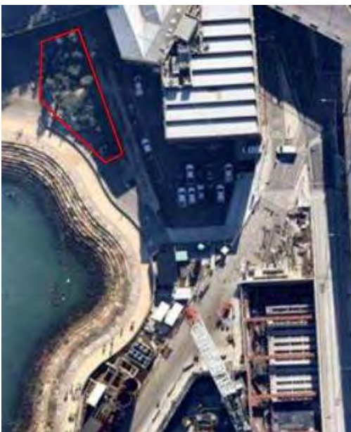
Figure 1 Bond Store and adjacent trees
