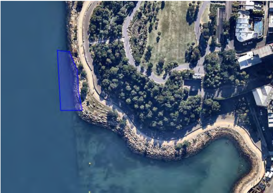
Figure 3 Nawi Cove Headland - Location of cooling water pipework existing in Sydney Harbour
