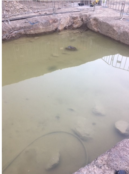
The effects of an effective flocculant on extremely turbid water.
