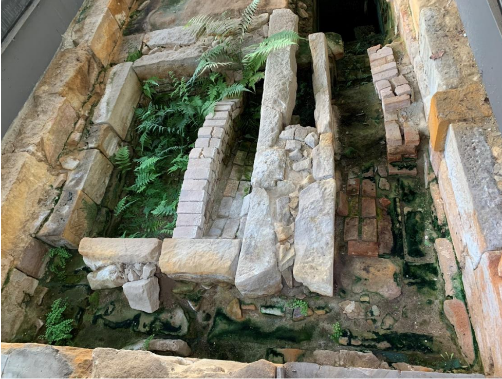
Plate 6: Parramatta Justice Precinct- Kitchen Pavilion, showing biological growth
