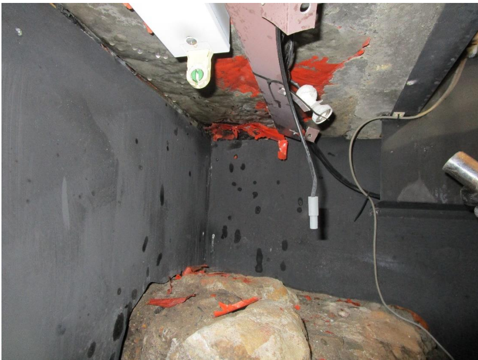
Plate 15: First Government House at Museum of Sydney –showing dripping of water onto archaeological remains and deterioration of building plastics
