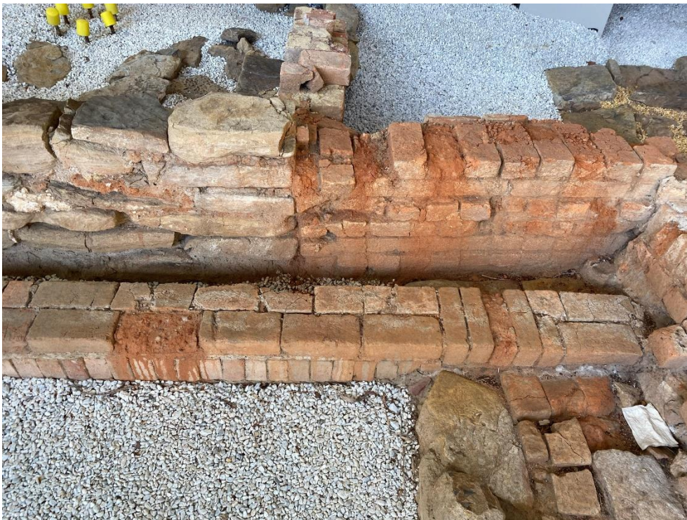
Plate 11: Early convict settlement at V by Crown, Parramatta – showing erosion from water ingress
