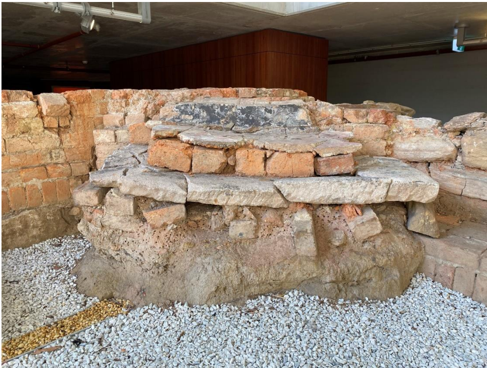
Plate 9: Early convict settlement at V by Crown, Parramatta – showing damage to mortar by native wasps
