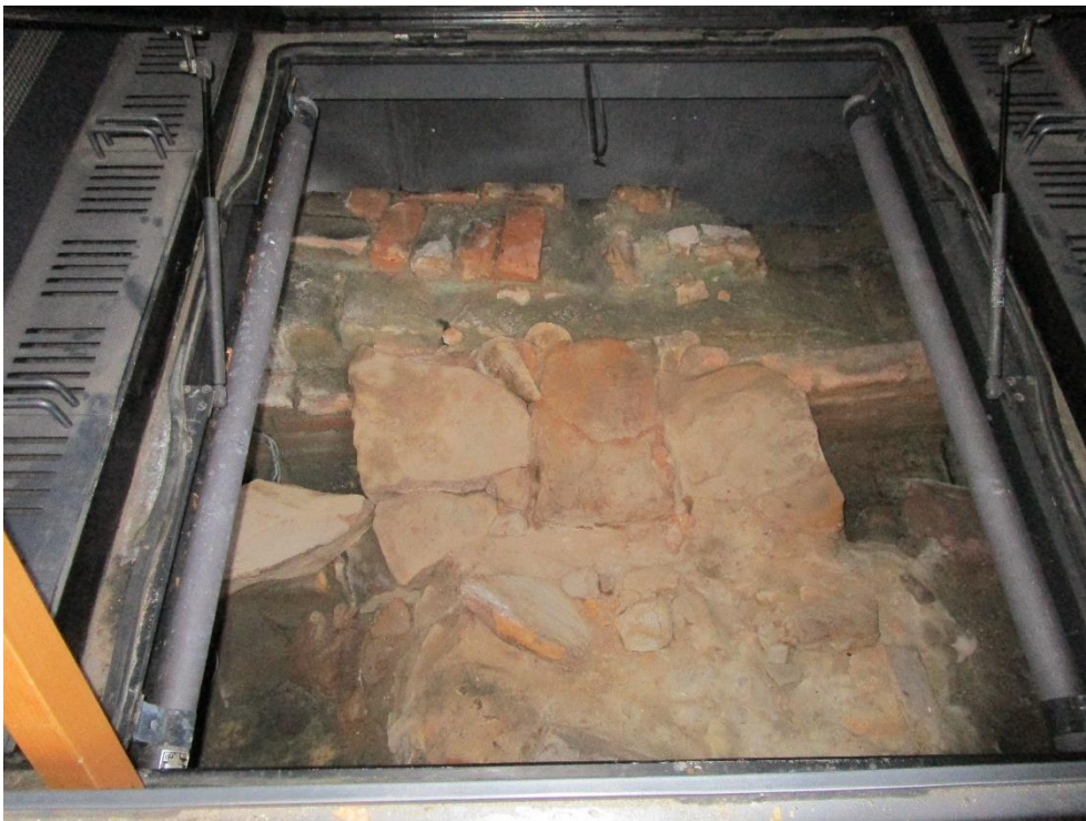
Plate 13: First Government House at Museum of Sydney – view within one of the windows, showing development of green/grey biological growth along top
