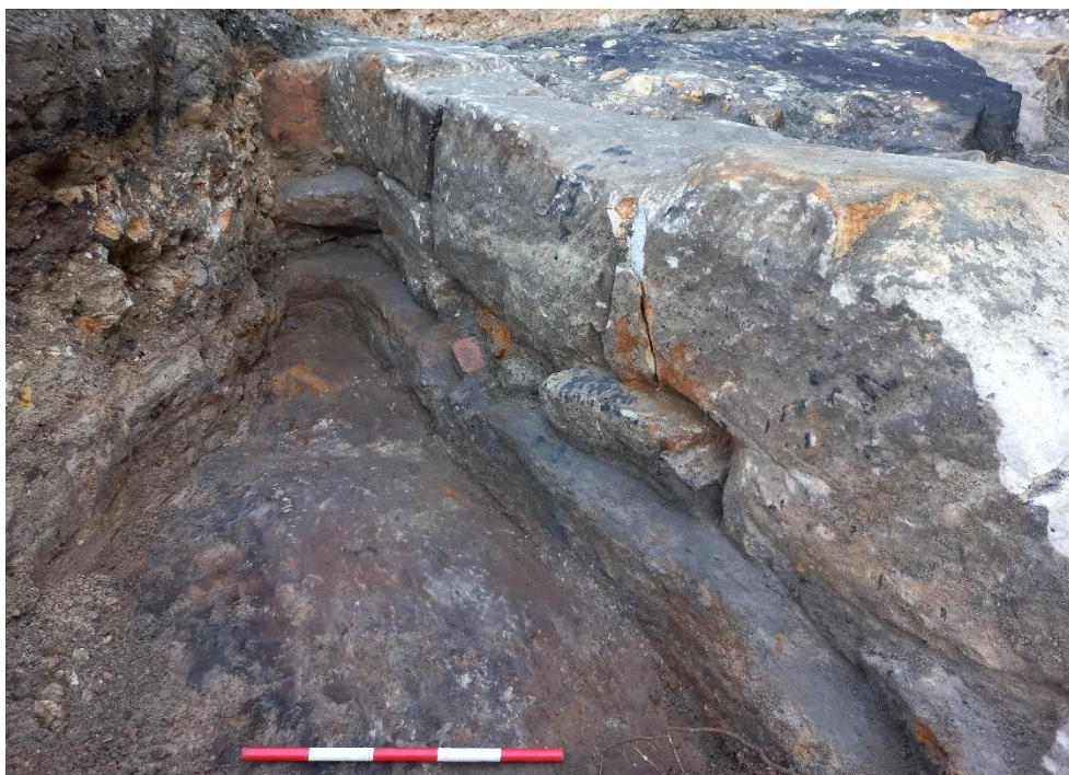
Figure 4.46: The cut down bedrock can be seen here below the wall. A thin brown organic skin has developed on the sandstone below. Scale 500mm. View to the north.
