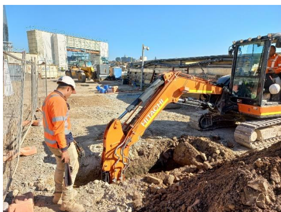
Figure 4.38: Excavation of Test pit 3 looking south.
