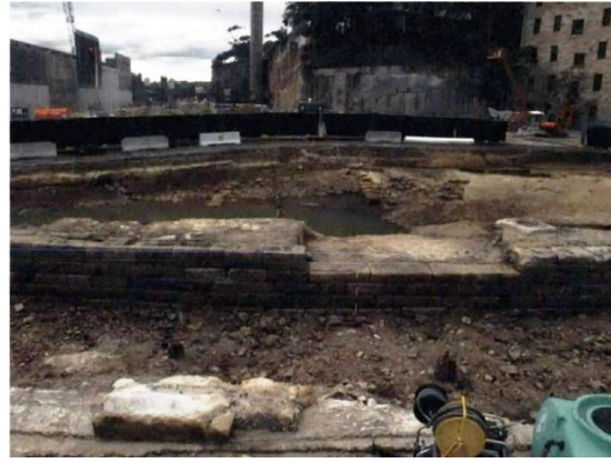
Figure 3.6: Dibbs' seawall looking northeast towards Dalgety stores (Austral Archaeology, 2016, p. 99)
