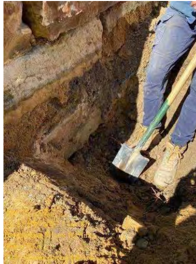
Figure 4: Concrete footing beneath sandstone blocks
