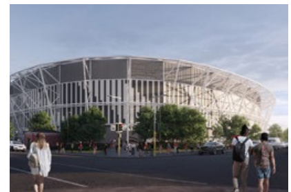
- Te Kaha Multi-Use Arena, NZ. Our QLD/NZ team continues to demonstrate unrivalled stadium expertise.
