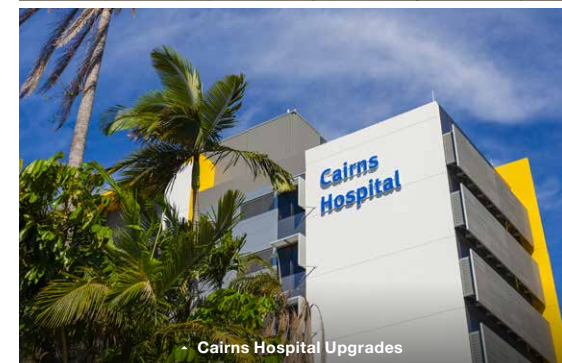
Cairns Hospital Upgrades
