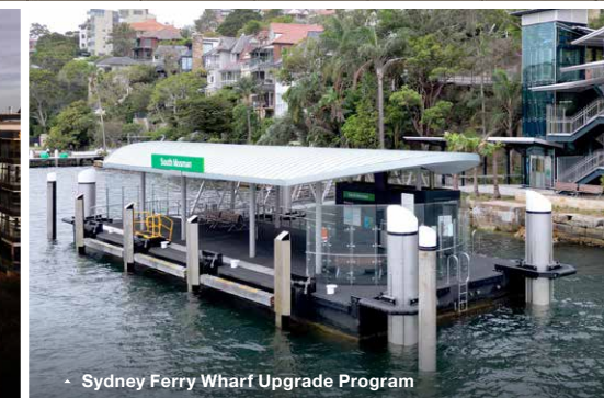
Sydney Ferry Wharf Upgrade Program
