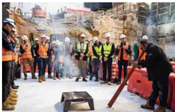
▴ Indigenous smoking ceremony at a BESIX Watpac project site - held within a designated safety exclusion zone with all works ceased.
