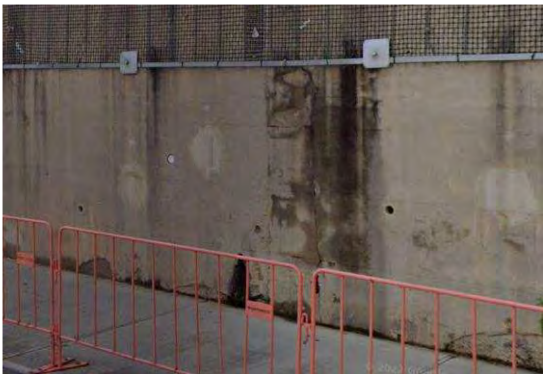
Figure 7: Cracking at the location of SBR 3.2.
