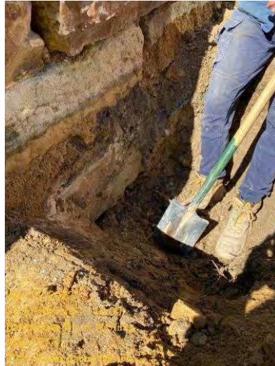
Figure 4: Concrete footing beneath sandstone blocks
