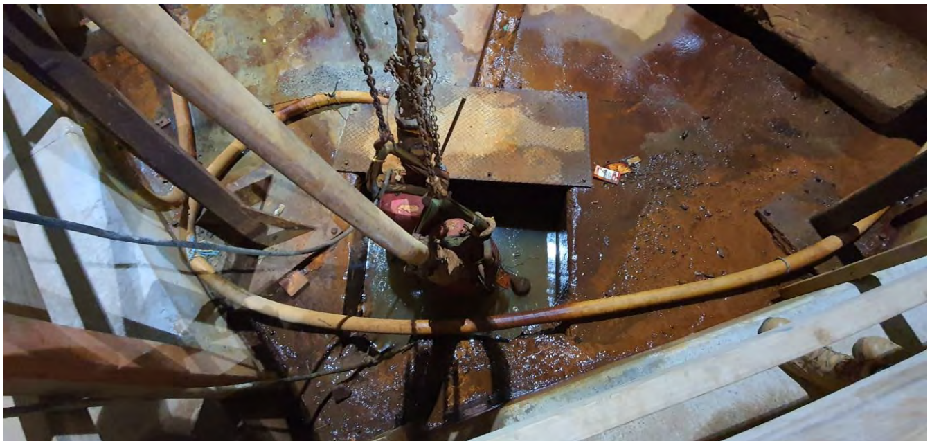
Figure 3 Dewatering Sump Pit & Pump in the Northern Shaft Basement 6 (GR-1)
